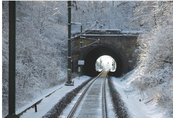
Gölshausen tunnel, the track was moved to the center for electrification
