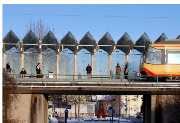
New station "Bretten Stadtmitte"
